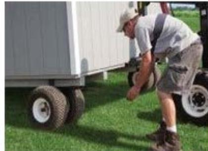
The dolly wheels are then placed, sliding easily into position.
